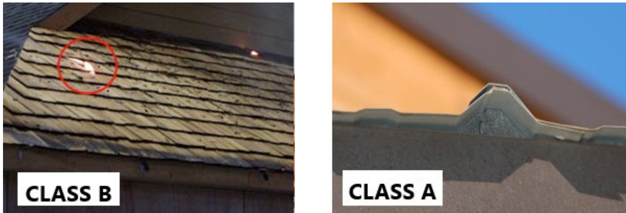
Figure 6.2. Examples of an untreated wood shake roof (Class B) that can accumulate flammable debris (left) and less-ignitable metal roof filled with noncombustible insulation (Class A) (right).
